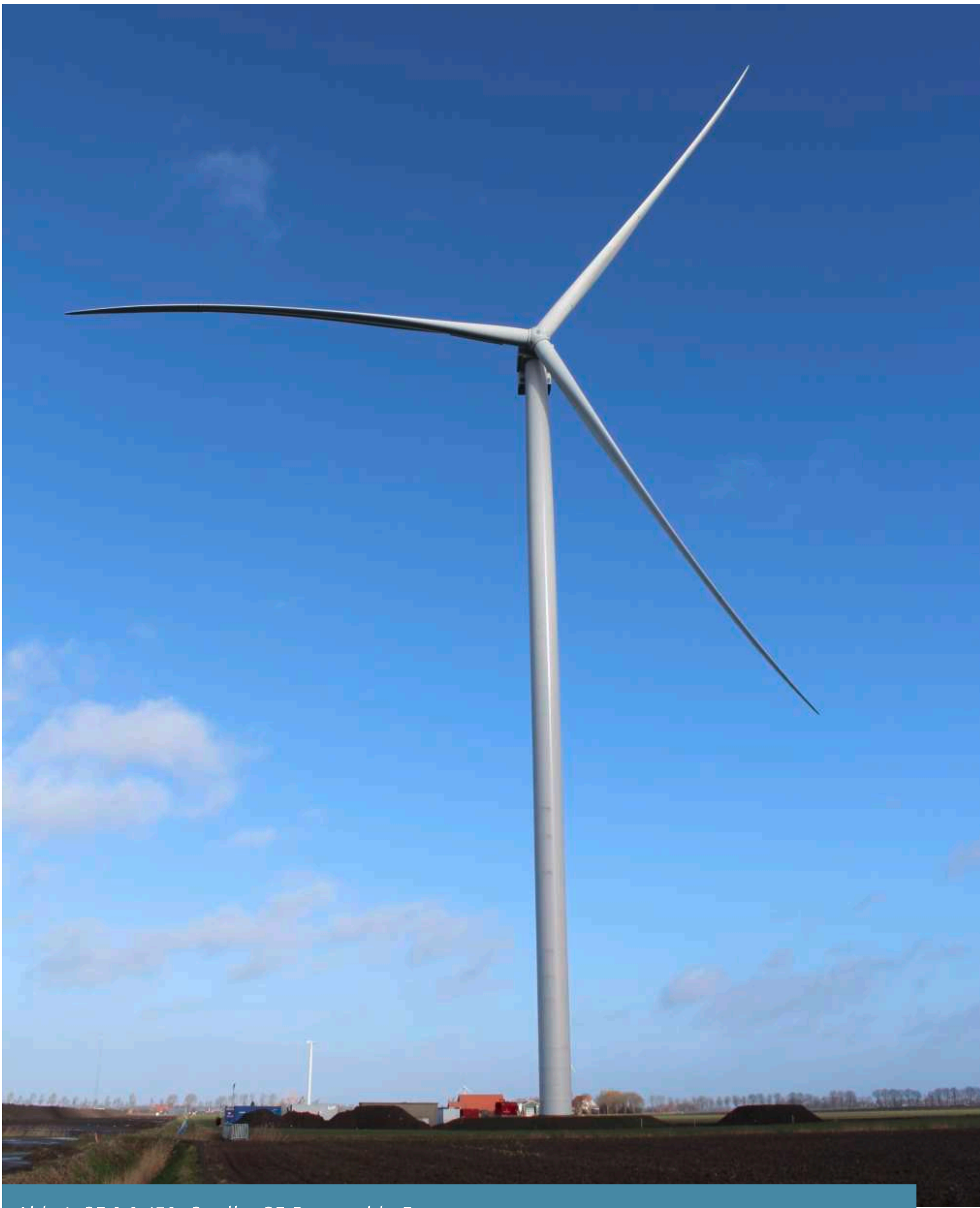
Abb. 1: GE 3.2-158. Quelle: GE Renewable Energy.
